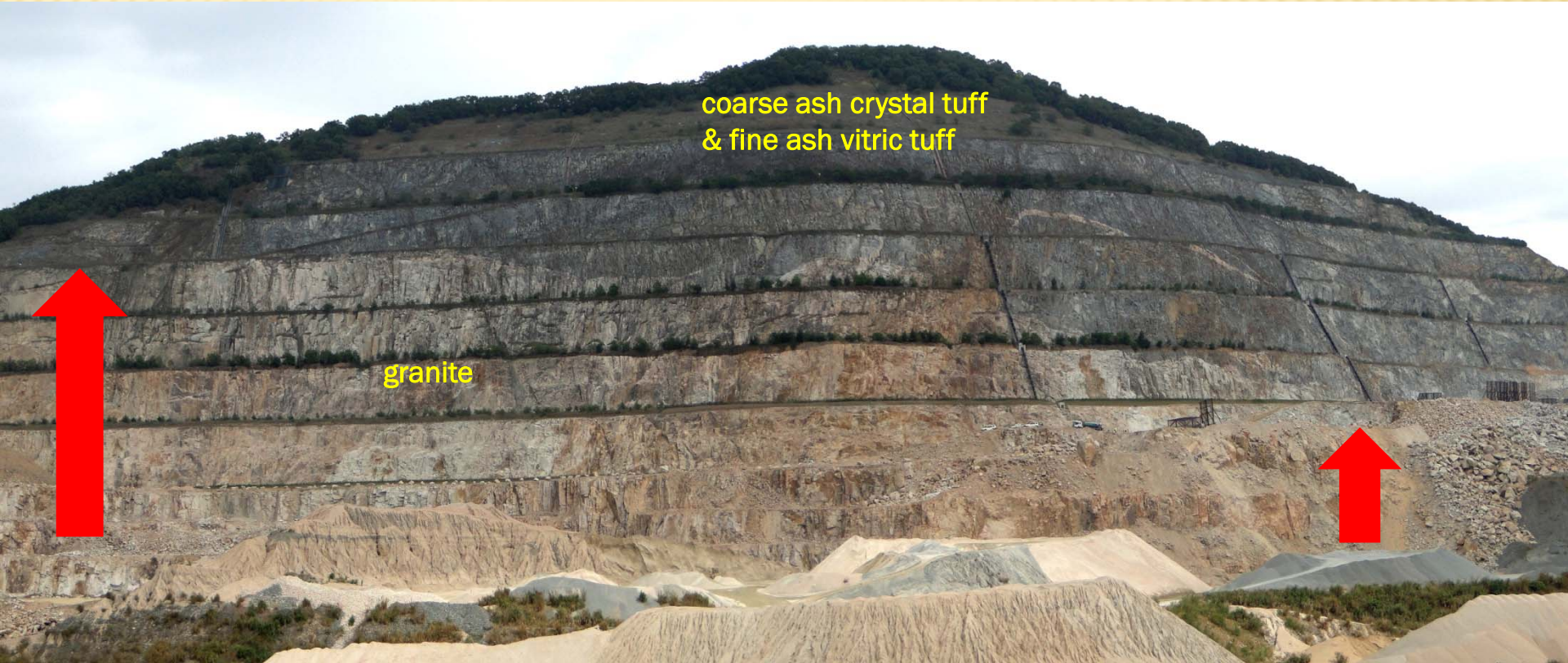
Front View of ARQ Rock Cut Slopes
